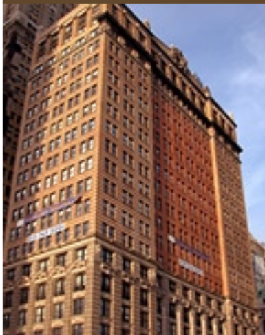
Battery @ 1 West Street
